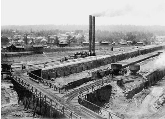
Tennessee Coal, Iron & Railroad coke ovens at the Pratt Mines near Birmingham, Alabama.
