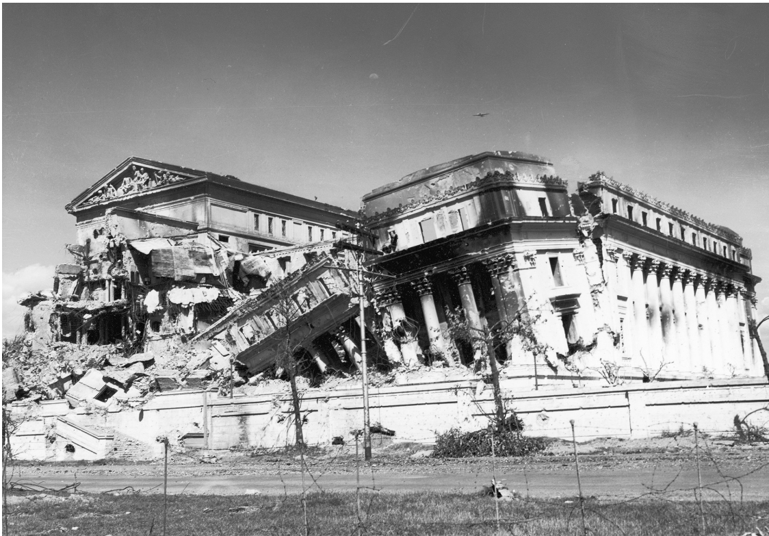
Juan Arellano's Legislative Building after two hours of point-blank shelling by the 37th Infantry Division
