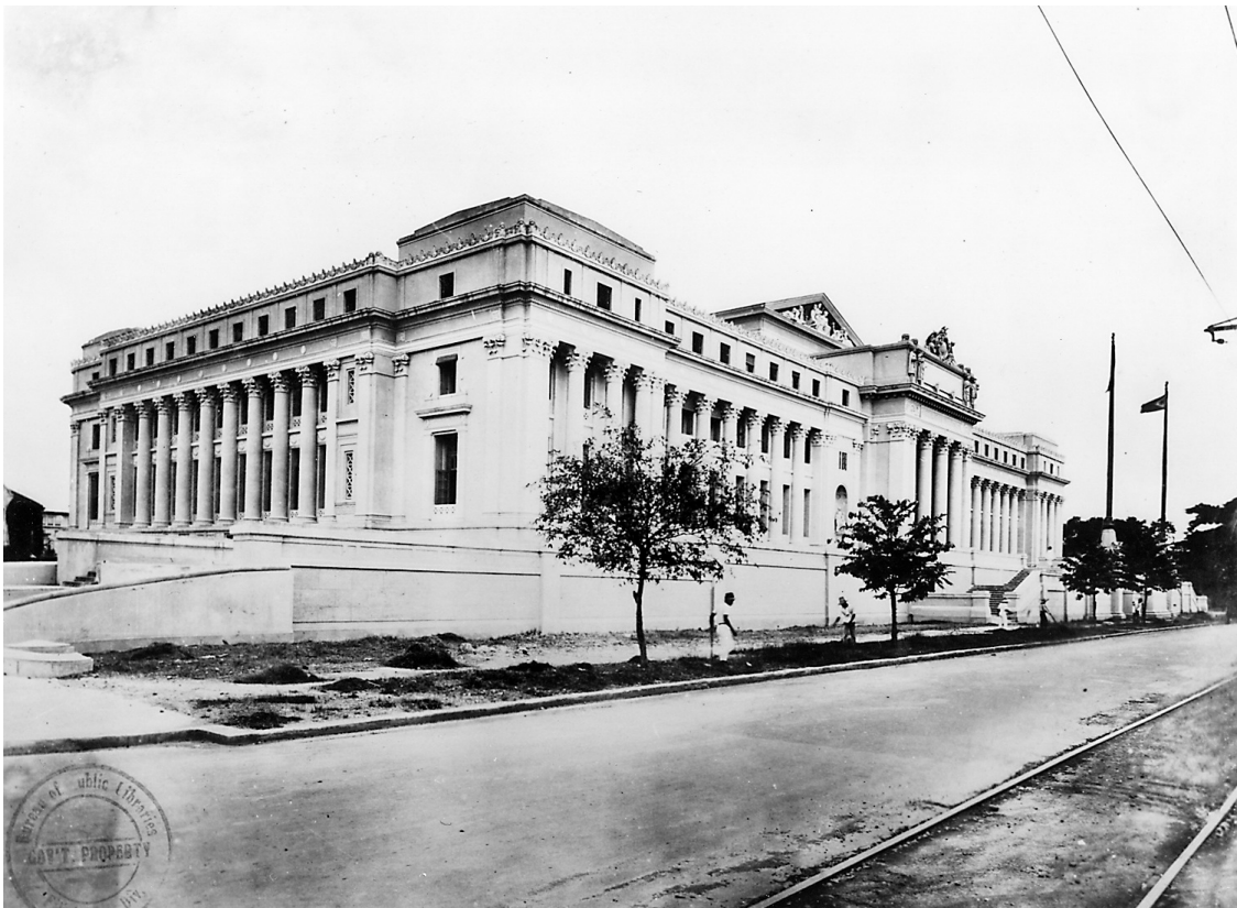
Juan Arellano's Legislative Building, completed 1926
