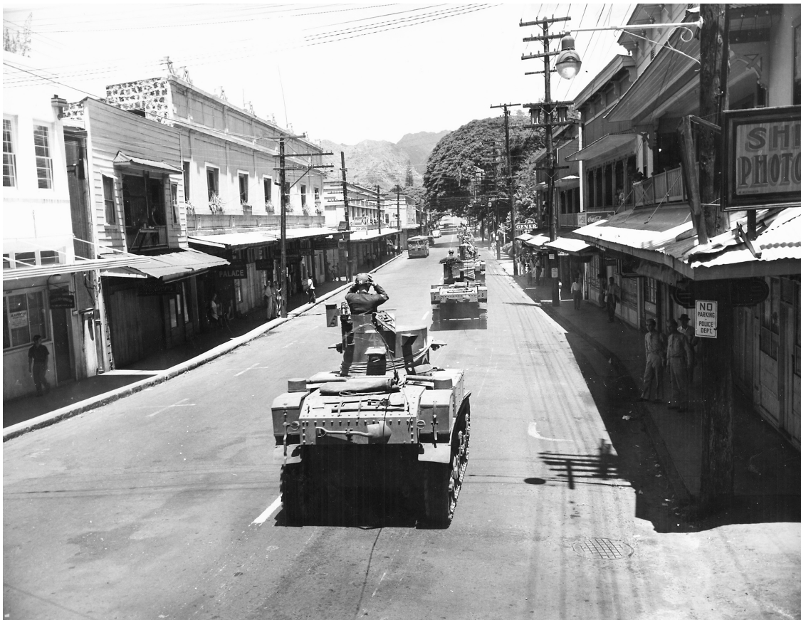
Tanks on Beretania Street in Honolulu during Hawai‘i’s nearly three years of martial law
