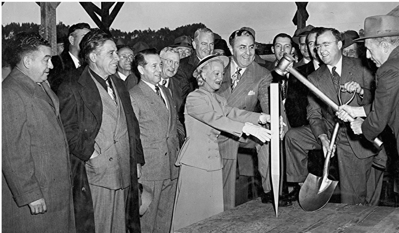
Daly City, California, 1949. FHA district director D. C. McGinness drives a spike to inaugurate construction of a shopping center, part of the segregated Westlake housing development.
